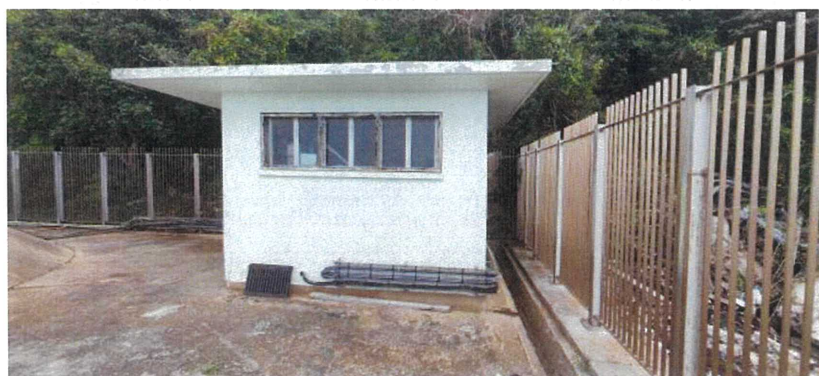
Figure 14: DSD technical room.
